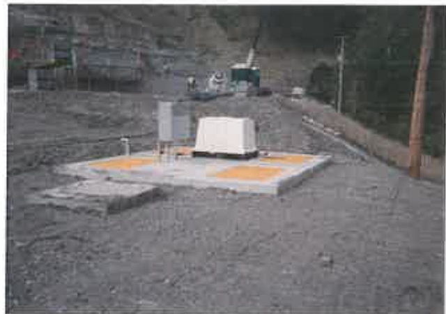
Equalization Tank/Pump Station During Construction
