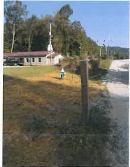
Fire Hydrant at Church
