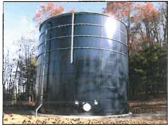
402,000-Gallon Water Storage Tank
