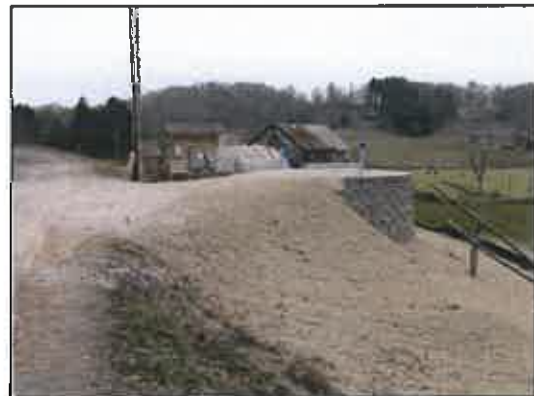
50 GPM Booster Station
