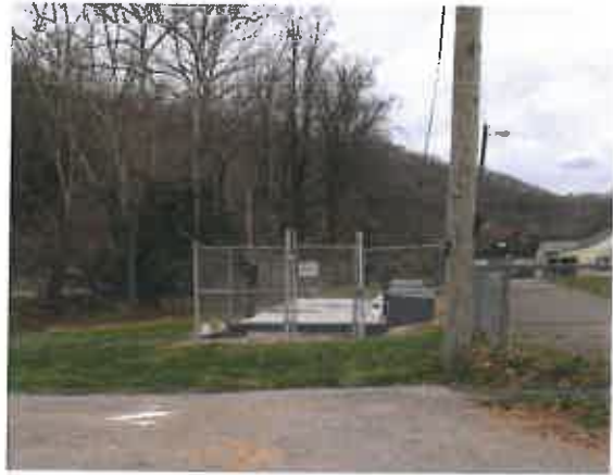
Existing Package WWTP to be Abandoned
