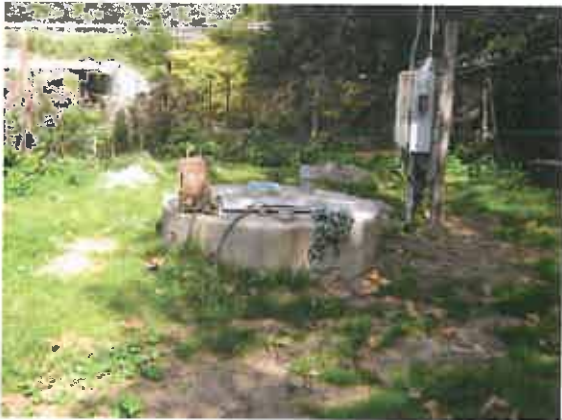
Before: Upper Drive Lift Station
