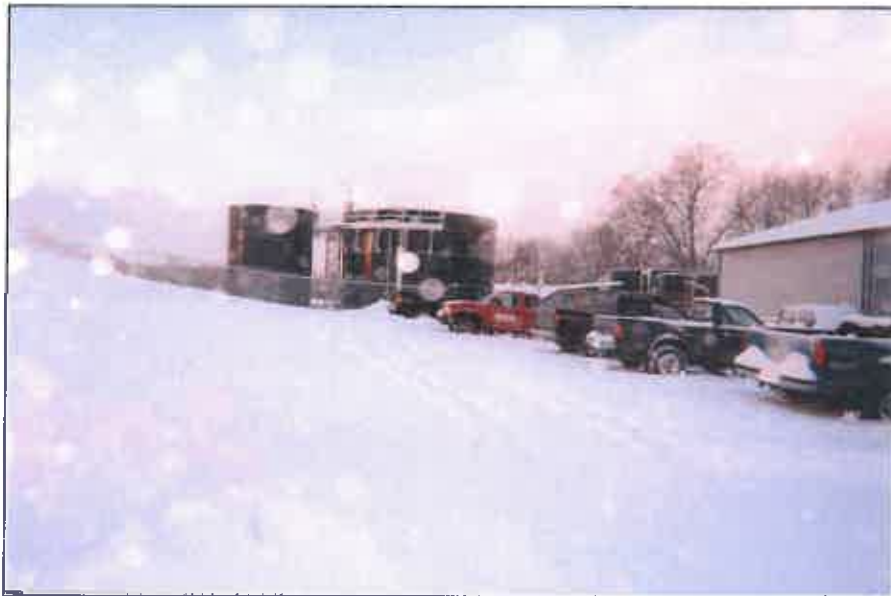
Aerobic Digester Tank (Left) and SBR Tank (Right)
