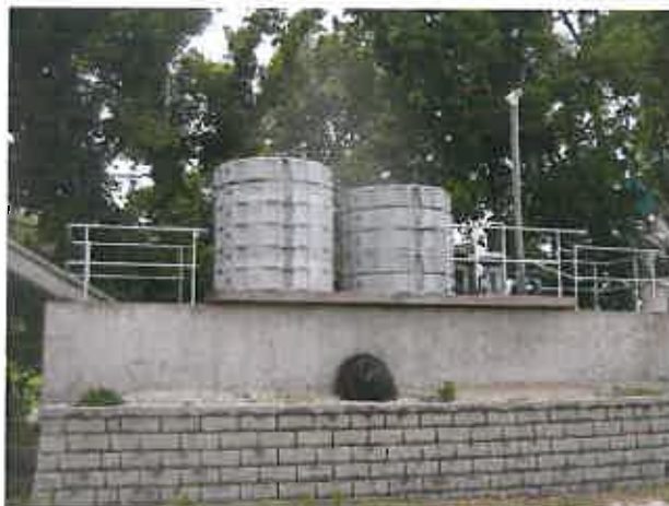
“Headworks” Facility with Scrubber Unit
