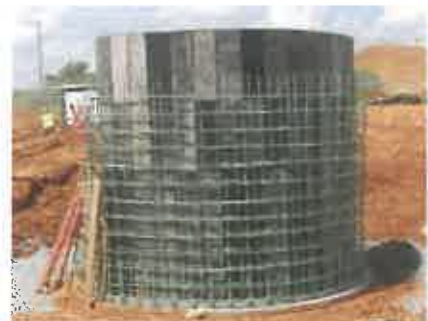
Charles Town Water Treatment Plant
