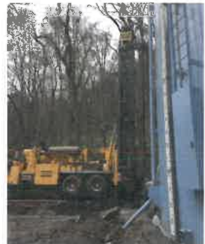
Frankfort Public Service District
