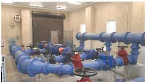
Charles Town Water Treatment Plant
