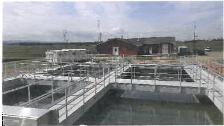
Charles Town Water Treatment Plant
