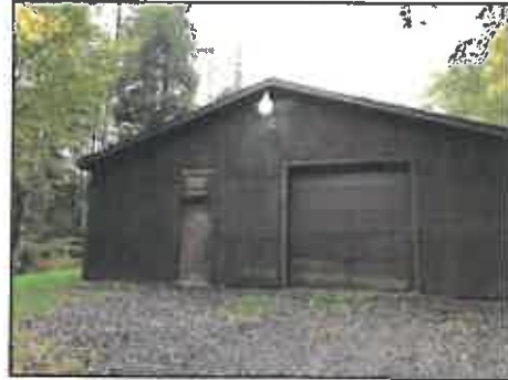
Old Cabin Treatment Plant
