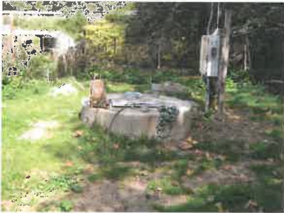
Before: Upper Drive Lift Station
