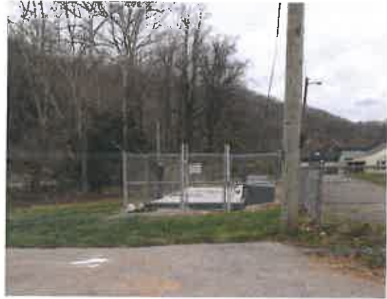
Existing Package WWTP to be Abandoned
