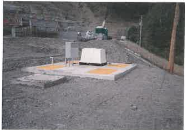
Equalization Tank/Pump Station During Construction
