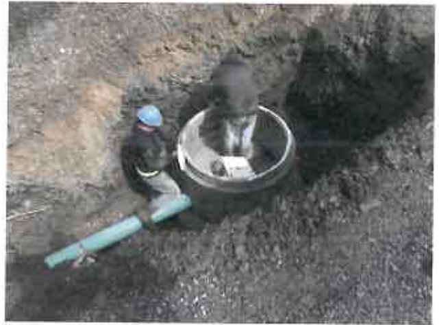
Town of Oakland – Sewer System Replacement
