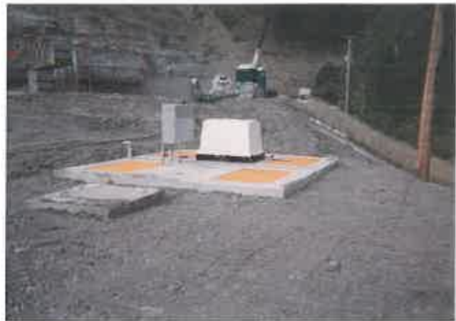
Equalization Tank/Pump Station During Construction
