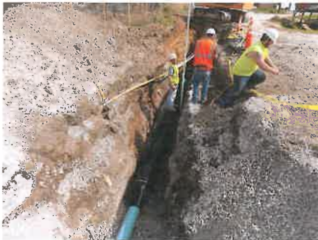
Sanitary Sewer Line Encasement at Water Line Crossing
