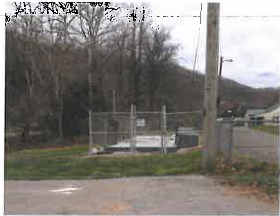
Existing Package WWTP to be Abandoned
