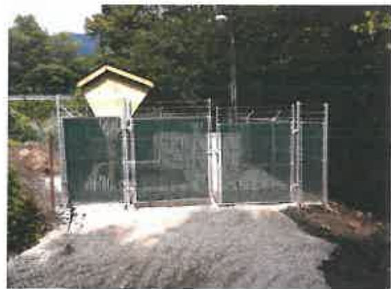
After: Upper Drive Lift Station
