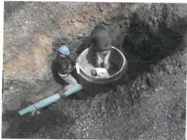
Town of Oakland – Sewer System Replacement
