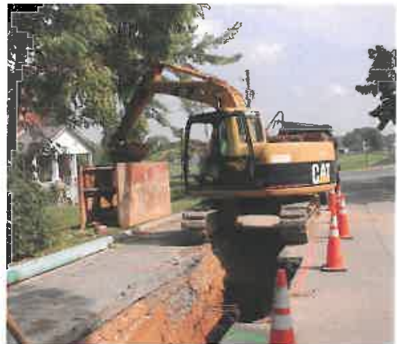
I&I Remediation - City of Waynesboro
