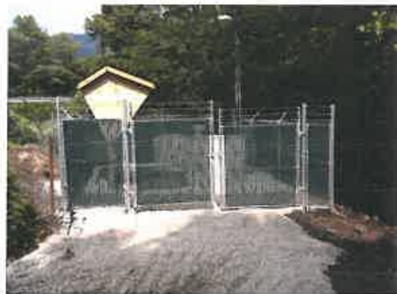
After: Upper Drive Lift Station
