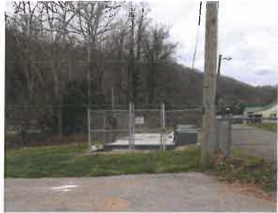
Existing Package WWTP to be Abandoned
