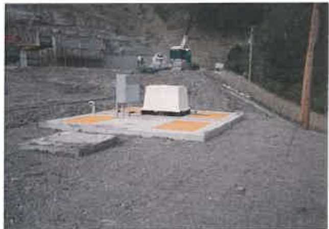
Equalization Tank/Pump Station During Construction
