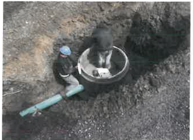
Town of Oakland – Sewer System Replacement
