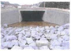
and construction observation and testing for the project consisting of demolishing and replacing the existing deteriorating concrete deck lid, repair spalling and cracking areas of existing sidewalls, and installation of a 8" diameter sanitary stub into the existing main line.
