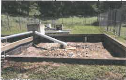
Comminuter at Lodge (above), and, sand filters (below, center) and polishing pond (below, bottom) at Ski Area of the Canaan Valley Resort State Park; Photos by Dunn Engineers Inc., taken during 2016 project for the DNR to assess wastewater treatment facilities at the park (Report is in Appendix C of this proposal)
