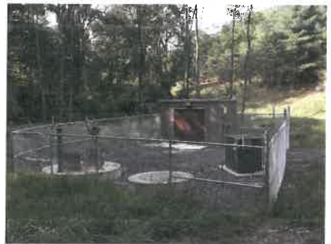
Frankfort PSD – Regional Sewer System
