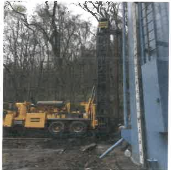
Frankfort Public Service District
