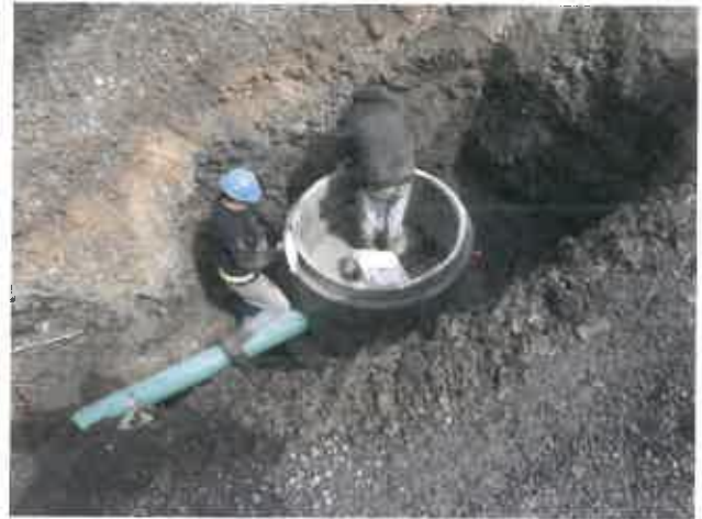
Town of Oakland – Sewer System Replacement
