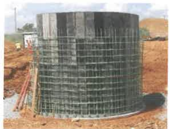
Charles Town Water Treatment Plant
