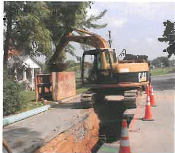
I&I Remediation - City of Waynesboro
