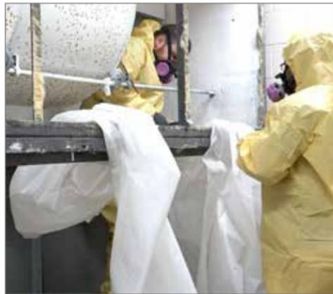
Depending on where the AHU is located we choose and deploy the specific equipment required for job. Then, as a licensed mechanical contractor we shut down the unit following all lockout and tag-out procedures. If the AHU is located in a Mechanical Room a containment area is established to prevent steam and moisture from affecting the indoor environment. Next, all electrical components and ducts are masked to keep them dry.
