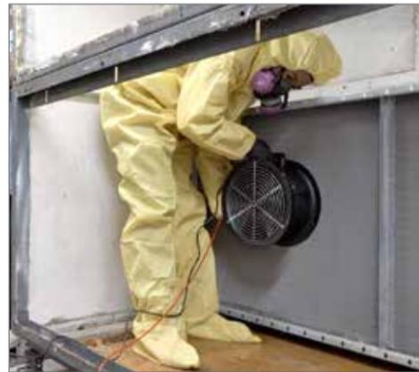
Pure Air Control Services Inc. performs their own proprietary Coil Cleanliness Verification Test (CCVT). This test is repeated across the span of the coils measuring the Delta P ( $\Delta P$ ) to determine which zones of the coil are most fouled. This is helpful to report the before state of the coil, as well as letting the tech know which areas of the coil will require the most attention. The data is logged and then cleaning commences.
