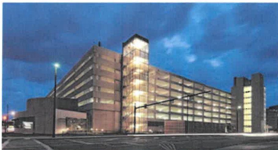
Cleveland Clinic Parking Garage Expansion Garage
