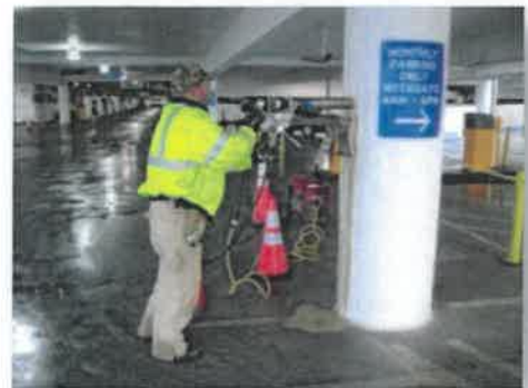
Figure 2 - Extraction of Concrete Cores from Parking Structure
