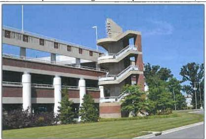
This vertical expansion project was needed to serve the growing airport passenger needs. The ramping system is a double helix arrangement utilizing one-way traffic and 70-degree parking. The structural system is cast-in-place, post-tensioned concrete to provide a large-span, open-feel parking and reduce long-term maintenance costs. The architecture includes precast architectural spandrel panels with brick inset and precast architectural column covers.
