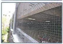
This 7-story, 2-bay, 489-space parking garage was developed to serve the growing on-campus population of the adjacent University of Maryland campus. The ramping system is a single-helix arrangement utilizing two-way traffic and 90-degree parking. The structural system is precast, prestressed concrete to provide quick erection, utilizing off site system production. The architecture includes brick, waterproofing painted coatings, and green screen.
