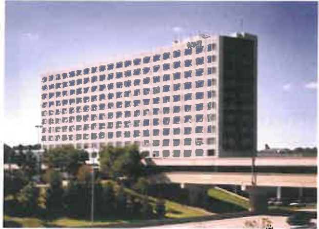
Hyatt Hotel at the Pittsburgh International Airport Dauphin County General Authority Pittsburgh, PA
