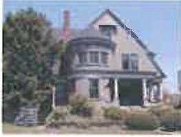
404 South Front Street (Harry C. and Jessie F. Franzheim House) Wheeling, WV (NRHP Reference #: 89000183) Customer: McKinley Architecture and Engineering Project Cost: $300,000
