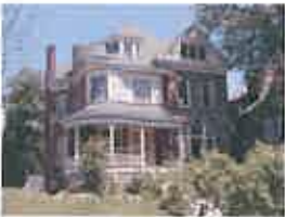
304 South Front Street Wheeling, WV (in Wheeling Island Historic District - NRHP#: 92000320) Customer: McKinley Architecture and Engineering Project Cost: $275,000
