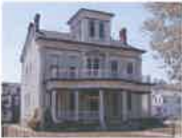
203 South Front Street (John McLure House) Wheeling, WV (NRHP Reference #: 91001013) Customer: McKinley Architecture and Engineering Project Cost: $300,000
