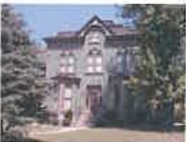
400 South Front Street Wheeling, WV (in Wheeling Island Historic District - NRHP#: 92000320) Customer: McKinley Architecture and Engineering Project Cost: $250,000
