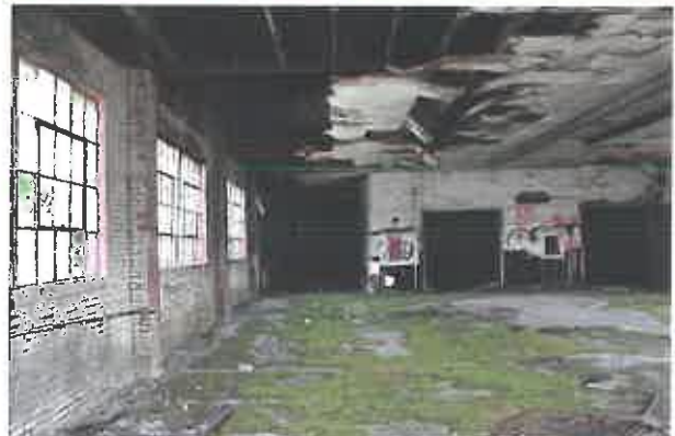
Right: Interior prior to renovation.
