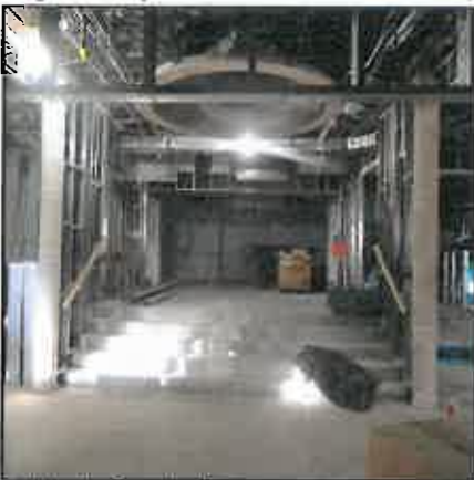
Lobby - In Construction
