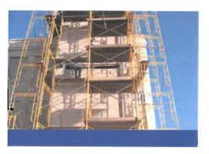
Exterior masonry of the elevator shaft was repaired where it was cracked and deteriorated.
