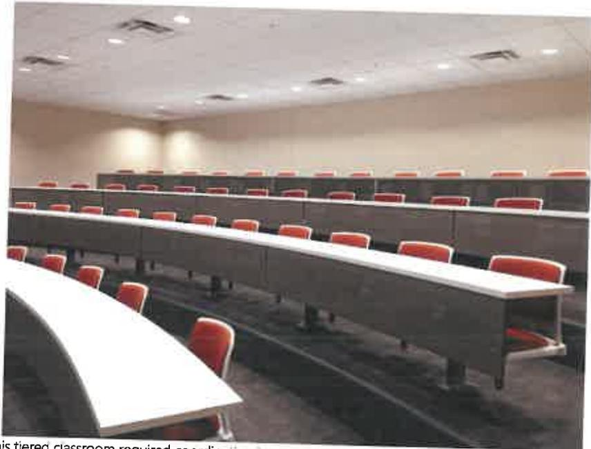
This tiered classroom required coordination between the furniture manufacturer and the contractor. Additional plywood was added to the stepped areas since the tables are directly attached to the floor, and the legs must also support the attached swivel chairs.
