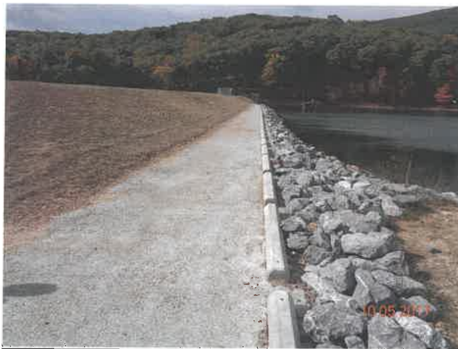
RESERVOIR DAM MODIFICATION, CACAPON STATE PARK (AFTER)
