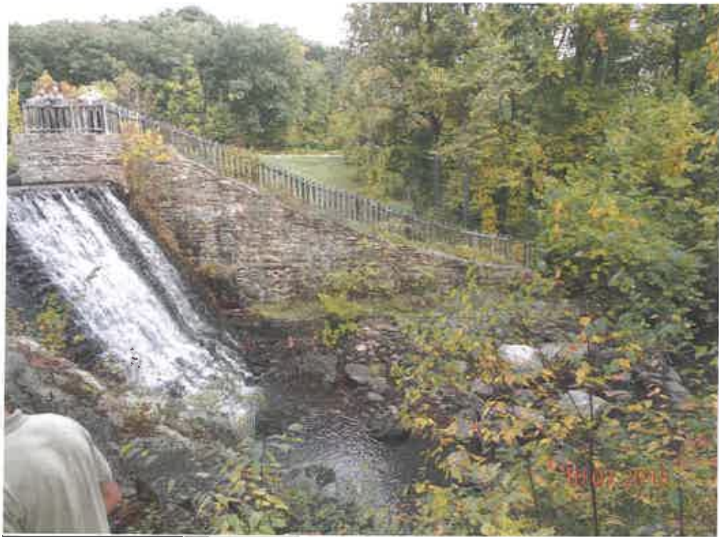
PARK DAM MODIFICATION (RCC), CACAPON STATE PARK (BEFORE)
