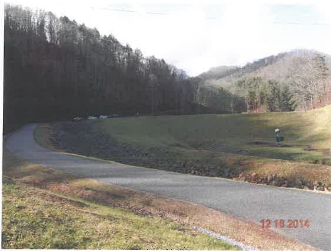
BERWIND DAM MODIFICATION (RCC), MCDOWELL COUNTY, WV
