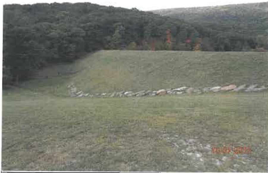
RESERVOIR DAM MODIFICATION, CACAPON STATE PARK (BEFORE)
