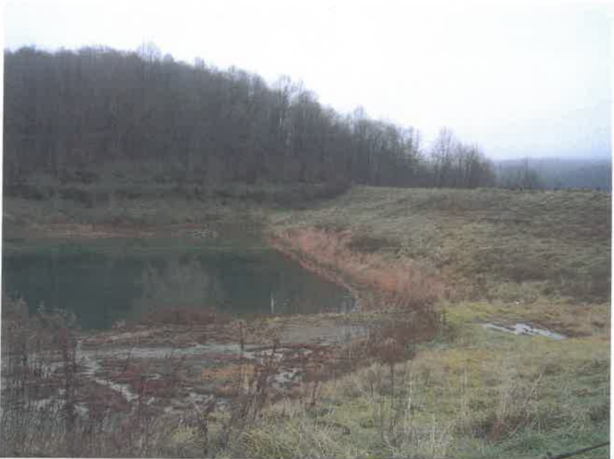
BAILEY DAM MODIFICATION, MONONGALIA CO., WV (BEFORE)
