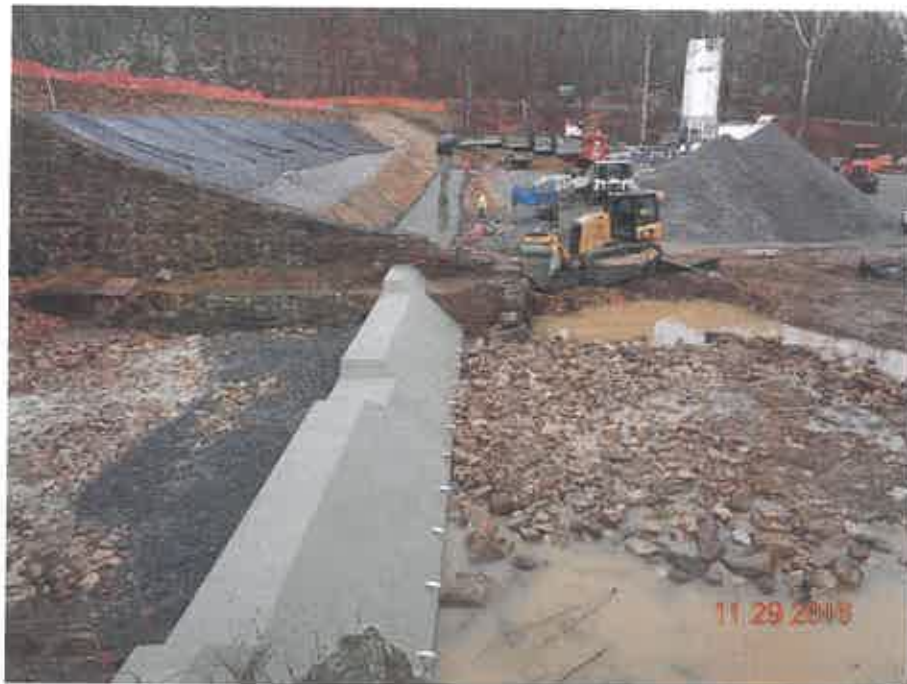
PARK DAM MODIFICATION (RCC PLACEMENT), CACAPON STATE PARK
