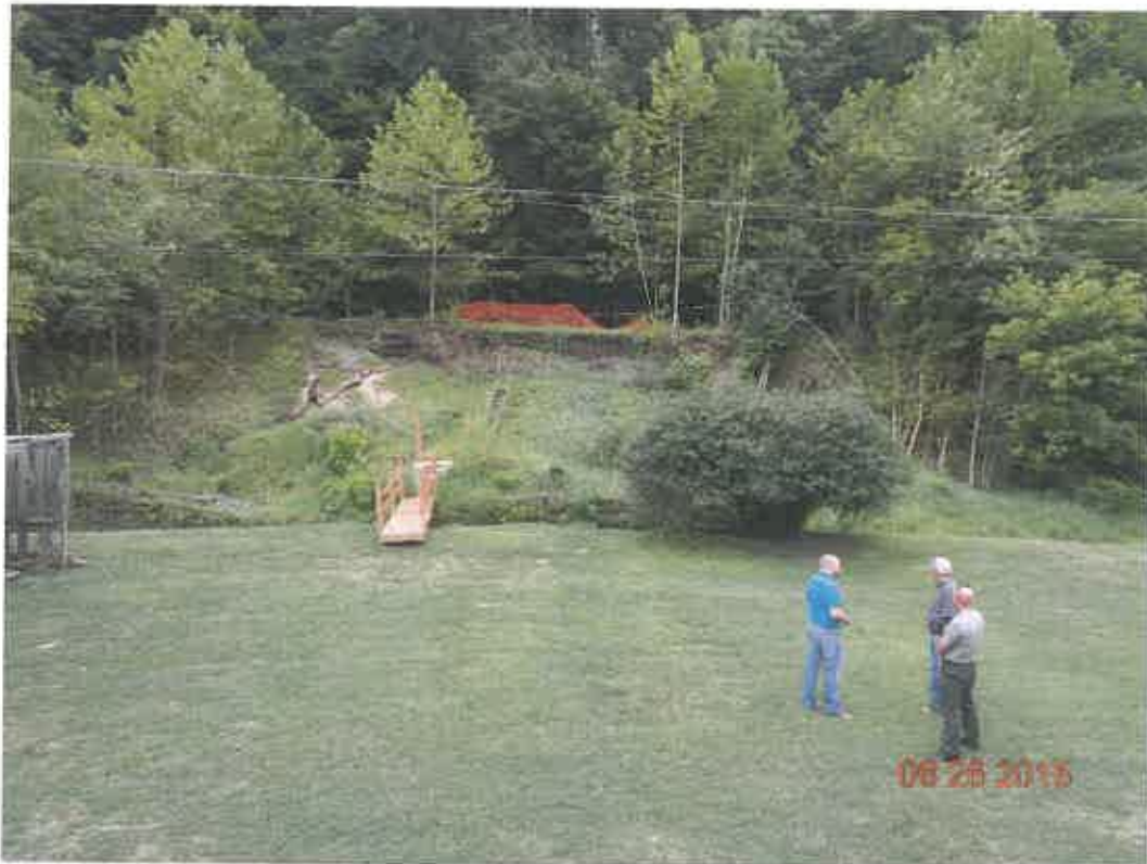
Overview of NBRT Landslide
