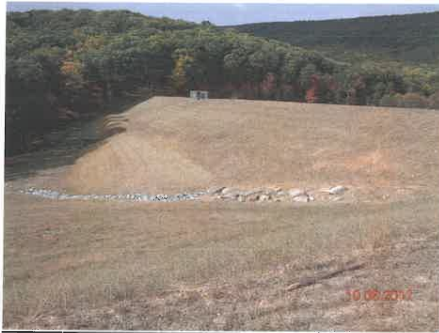
RESERVOIR DAM MODIFICATION, CACAPON STATE PARK (AFTER)
