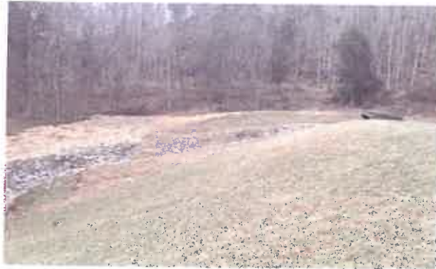
Cedar Lake Dam No. 2 Spillway
