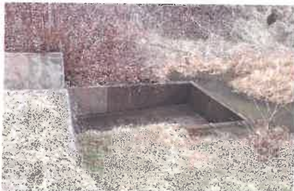
Cedar Lake Dam No. 1 Control Structure
