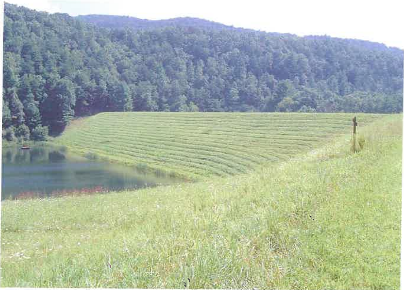
Todd Lake Dam (UNR 10) – Augusta County, VA
