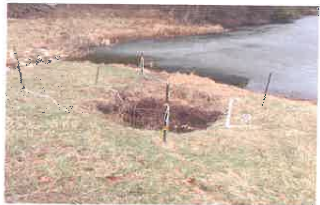
Cedar Lake Dam No. 2 Riser
