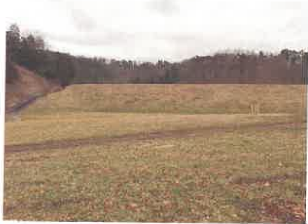
Cedar Lake Dam No. 1
