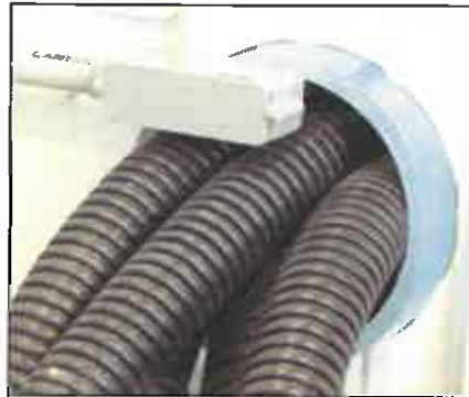
Ex 2: 8" diameter pipe for thru-wall hose run
