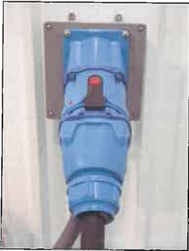
Truck Loading and Blending Skid Receptacle/Plug - 6" x 6" x 4" junction box shown with receptacle, receptacle housing & plug
