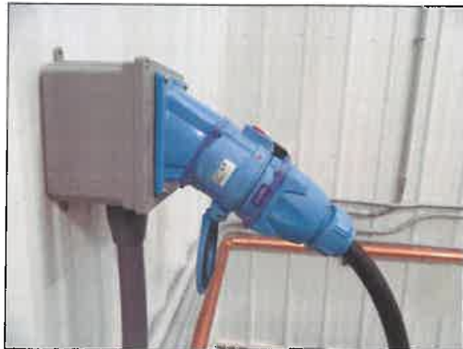
Truck Loading and Blending Skid Receptacle/Plug - 6" x 6" x 4" junction box shown with receptacle, receptacle housing & plug
