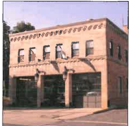
Central Fire Station
