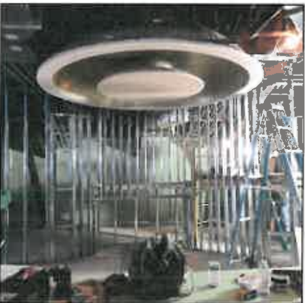
In-Progress Bar Area
