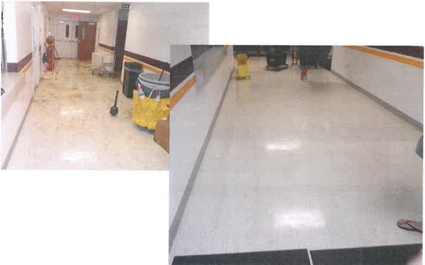
Flooding of Local School in Charleston, WV
