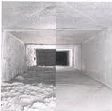
HVAC System Cleaning
