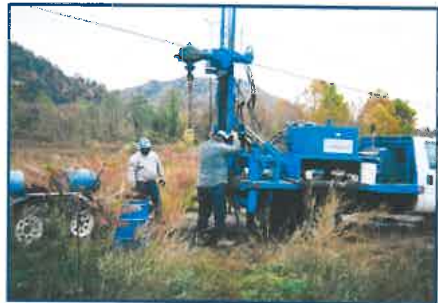
Environmental Sampling for an Underground Storage Tank Site Investigation
