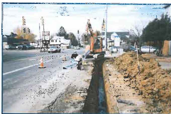
Replacement of Water Line along Route 60 near Ceredo, WV
