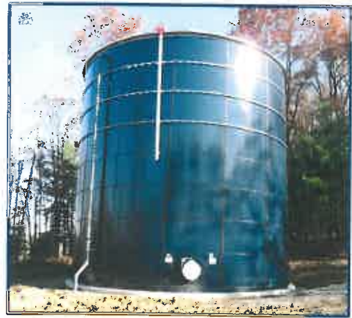
400,000 Gallon Water Storage Tank Near Philippi, WV
