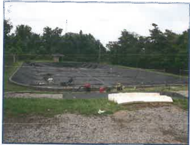
Water Storage Reservoir Floating Cover Replacement In Wellsburg, WV
