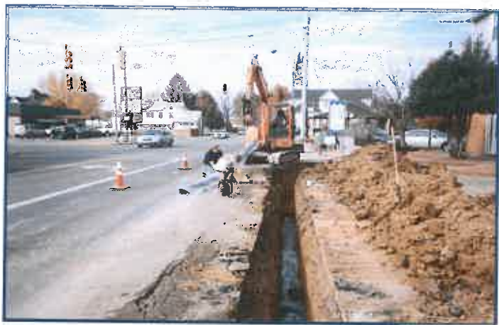
Replacement of Water Line along Route 60 near Ceredo, WV
