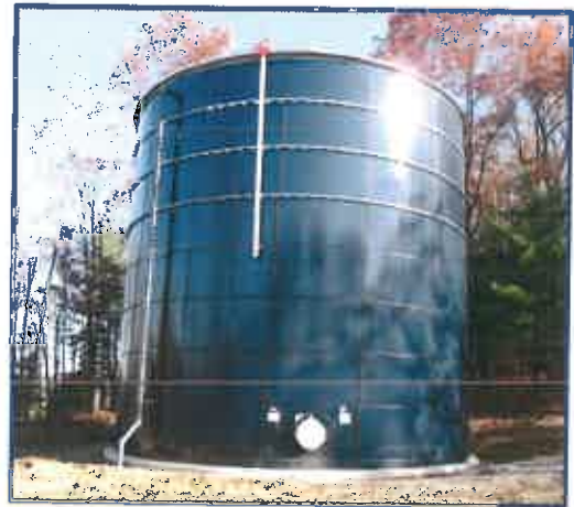
400,000 Gallon Water Storage Tank Near Phillippi, WV
