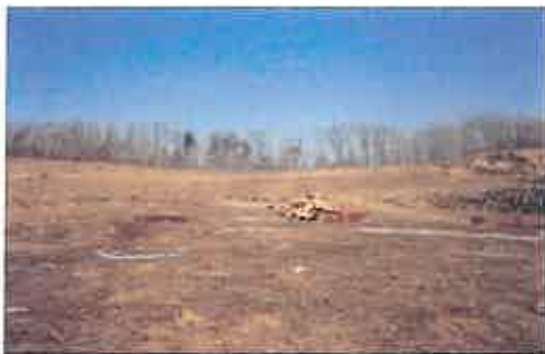
Prior to capping, the landfill area was poorly vegetated and experienced much erosion.
