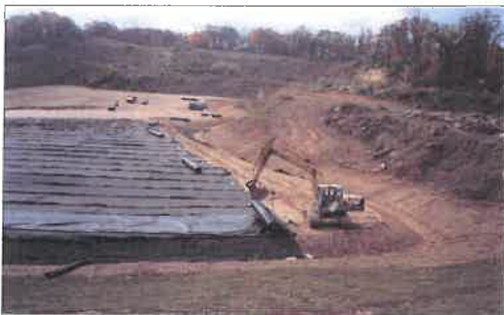
The project included construction of 19 acres of a geosynthetic cap system.
