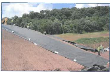
soil and placed. Historically the landfill construction has progressed as a series of benches (or lifts) which were capped once available airspace was exhausted. In this case, exhaustion of the landfill's active airspace was expected sometime during the year 2004. Expecting the exhaustion of the landfill's airspace, the Owner made the decision to expand, necessitating the implementation of phases of a multi-phased expansion.
