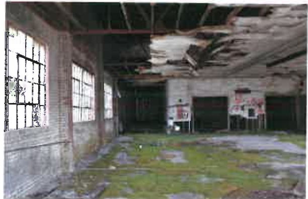
Right: Interior prior to renovation.
