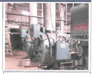
Morgantown High school, like others throughout the state, has seen many changes through the years. Previous upgrades shifted heating load away from the steam boiler plant, resulting in the plant being significantly oversized to the load and operating with low efficiency. The 40 year old boilers have exceeded their operational life and are experiencing reliability issues.
