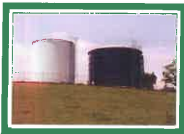
Alderson Water Storage Tanks
