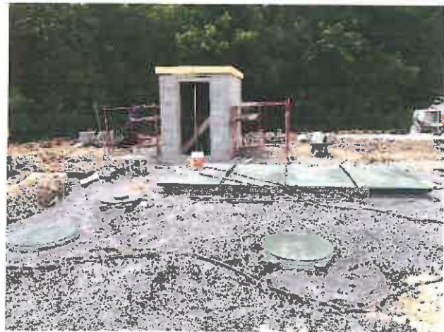
Installation of Orenco treatment units
