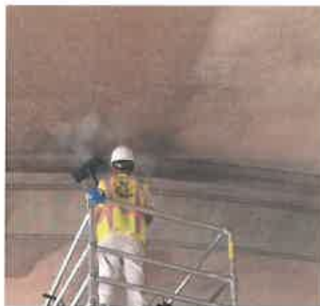
Sacramento Valley Train Station, Sacramento, CA
