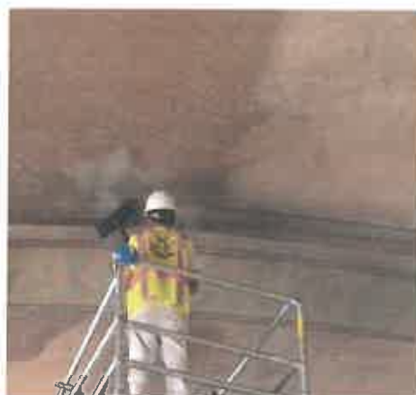
Sacramento Valley Train Station, Sacramento, CA
