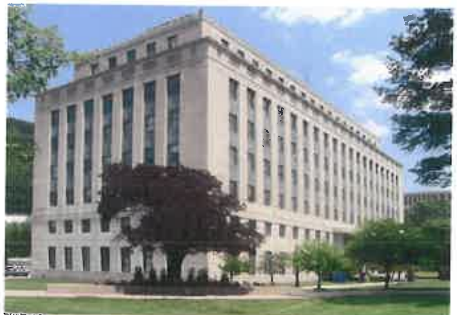
Building 3 Renovations included HVAC, fire safety, lighting, plumbing, indoor air quality and electrical power engineering.
