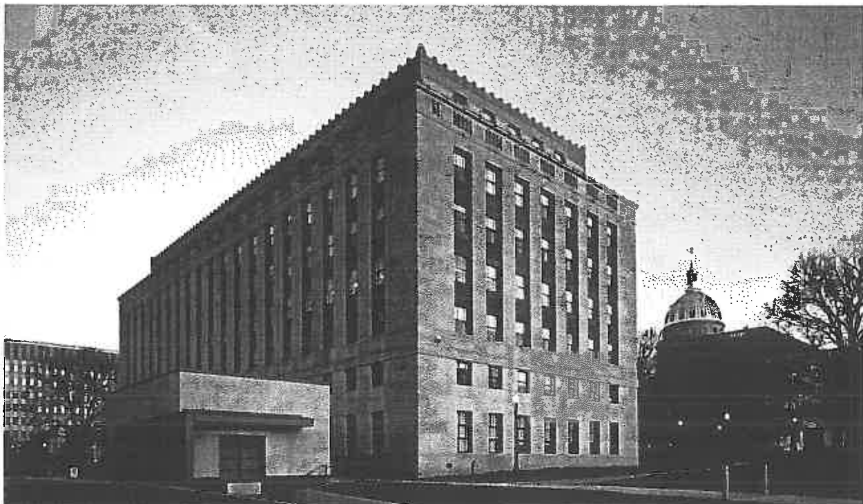
WV State Capitol Complex featuring the New Loading Pavilion at Building 3 which connect to the basement via a secure tunnel.
