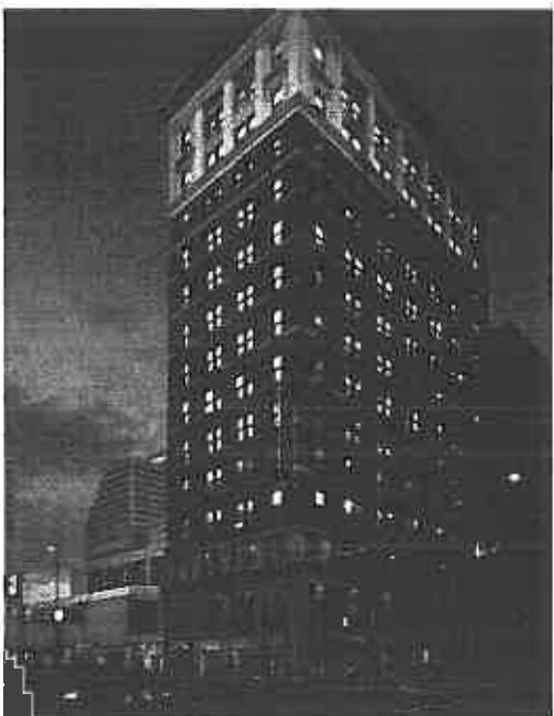
Project: Traction Building – Cincinnati, OH Professional Services: 2018-Present
