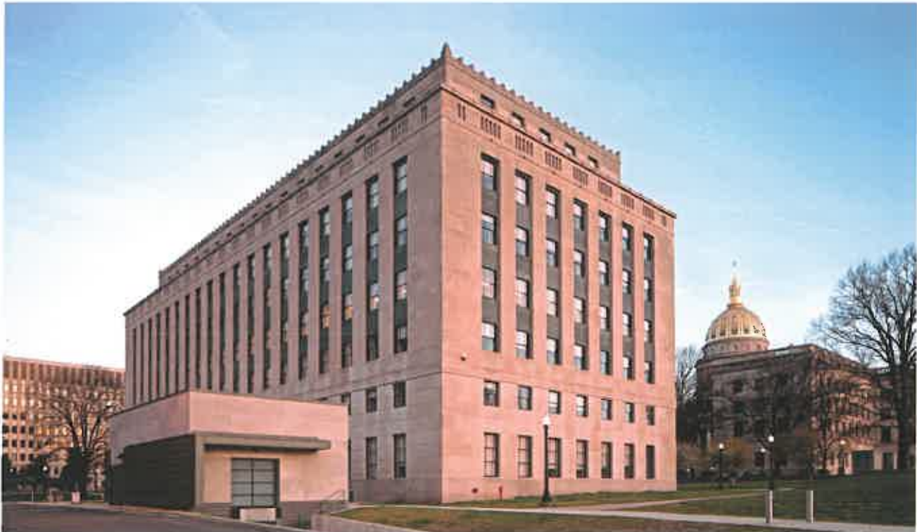
WV State Capitol Complex featuring the New Loading Pavillion at Building 3 which connect to the basement via a secure tunnel.
