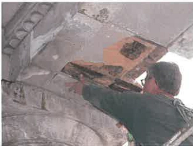
WWU Oglebay Hall facade investigation
