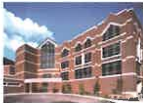
Project: Gallagher Student Center, Xavier University - Cincinnati, Ohio Client: Xavier University
