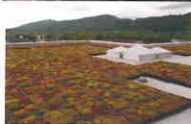
HRDC's Green Roof
