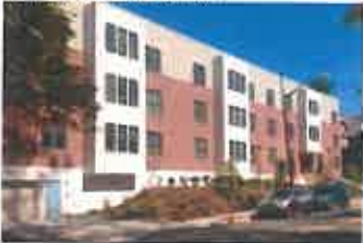
5637 Forbes Avenue Apartments
