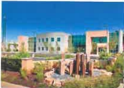
ALCOSAN customer service building
