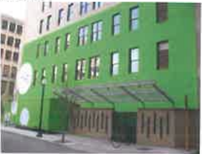
Century Building's Bike Station
