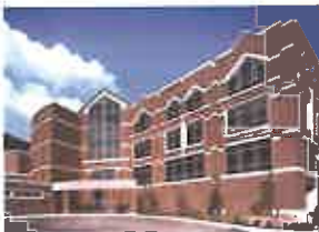
Project: Gallagher Student Center, Xavier University - Cincinnati, Ohio Client: Xavier University
