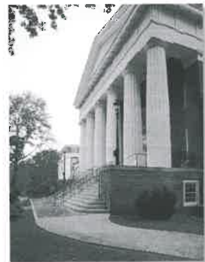
The Virginia School for the Deaf and Blind Staunton, VA Credit: Preservation Design Partnership, LLC
