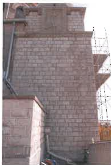
Limestone elevations repointed
