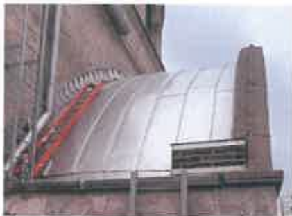
New standing seam metal roof
