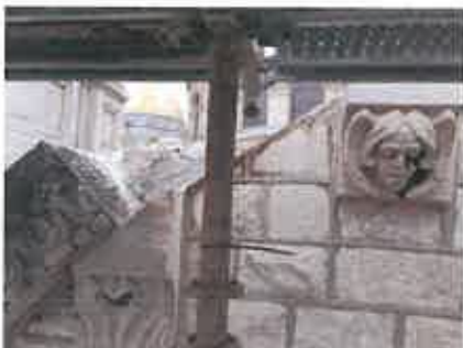
Rebuilding the Springfield Avenue parapet
