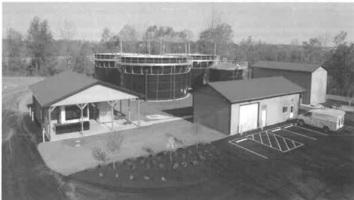
PNGI Charles Town Gaming LLC - Wastewater Treatment Facility
