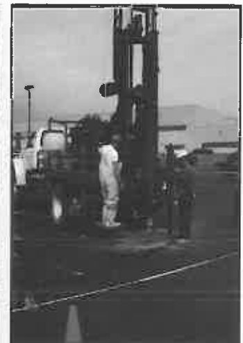
Drilling on Flat Terrain
