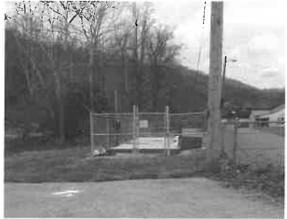
Existing Package WWTP to be Abandoned
