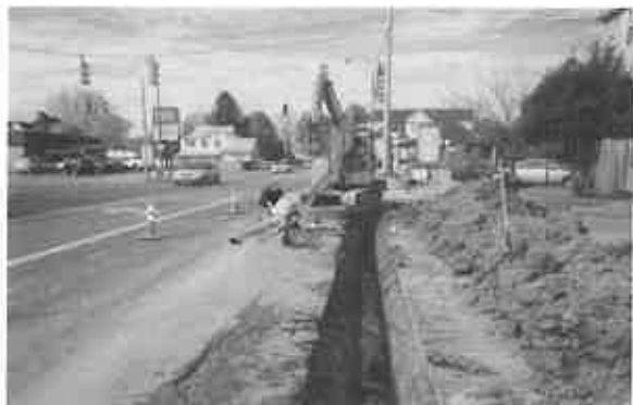
Replacement of water line along US Route 60.
