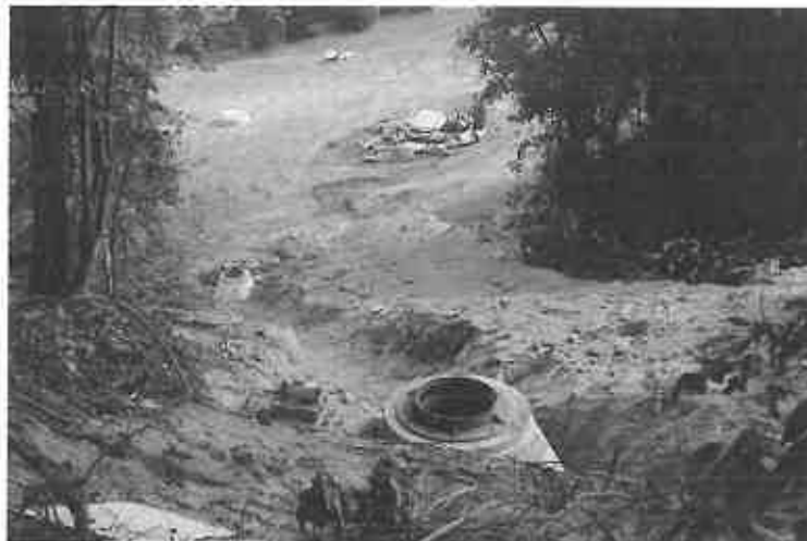
Manhole During Construction
