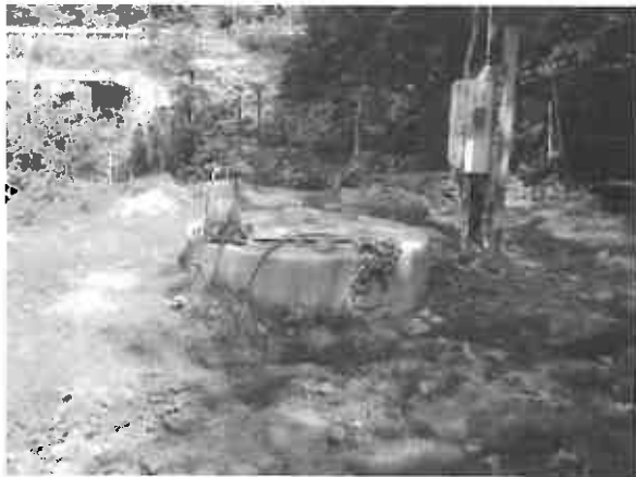
Before: Upper Drive Lift Station
