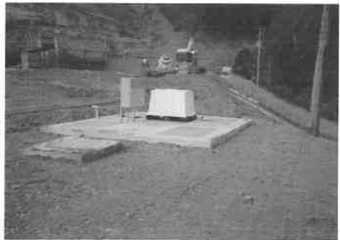
Equalization Tank/Pump Station During Construction
