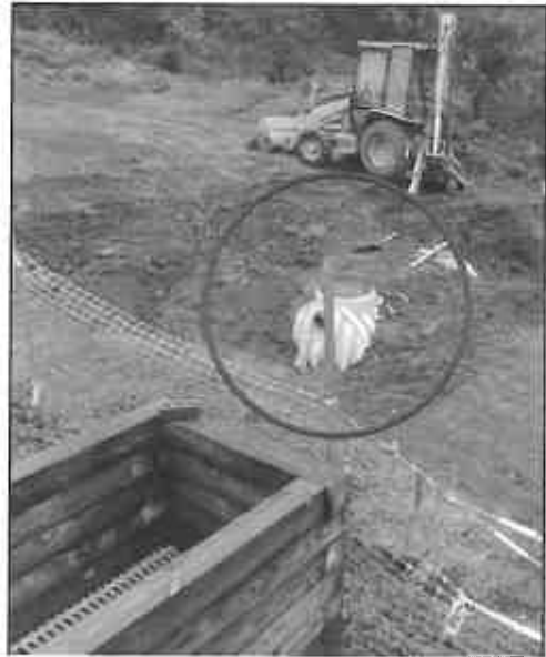
New Chlorine Contact Basin, Under Construction
