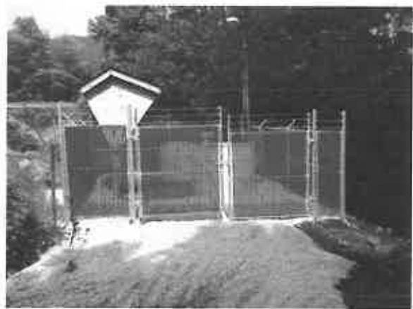
After: Upper Drive Lift Station
