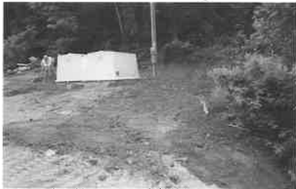
New booster station during construction.
