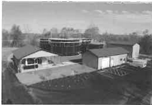
Wastewater treatment plant
