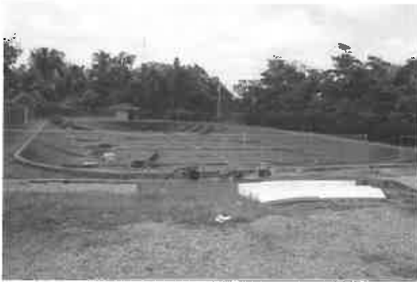
Reservoir Floating Cover Replacement
