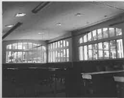
View Showing Both Natural Daylighting with Light Louvers, as well as Light from Bulbs
