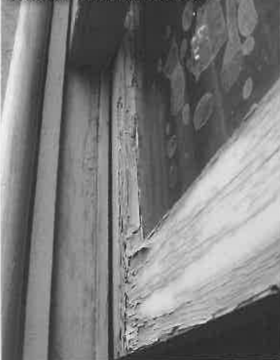
Exterior Window Before
