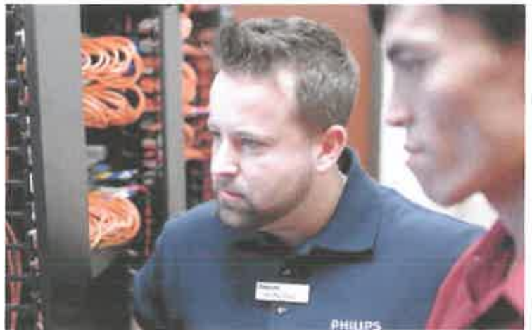
Bringing Value Added Services to the hospital server room.
