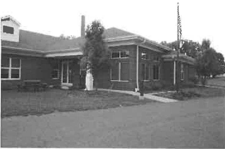
TURNING POINTE AT JACKIE WITHROW HOSPITAL Beckley, WV
