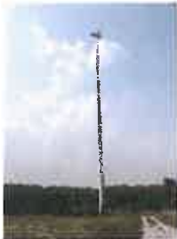
Cellular Tower Site Assessment
