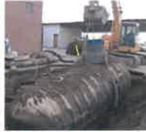
Underground Storage Tank Removal
